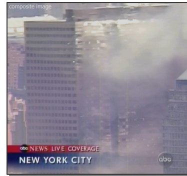
(Fig.2) A still image from the ABC News video shows no fire in WTC 7. It also shows a strange gash that runs all the way up its side.
