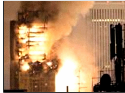
(Fig. 5) High-rise fires typically show dramatic flames spreading throughout the building.
