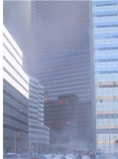
(Fig. 4) A photo of WTC 7's north face taken at 3 PM shows fires so small they are barely visible from outside of the enormous building.
