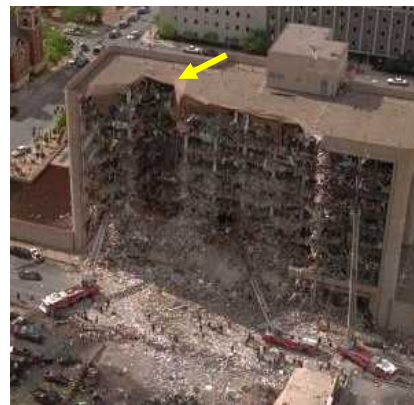
(Fig. 8) An aerial photo of the Murrah Building bombing shows a hollowed out vertical shaft (arrow) that runs up the entire height of the building, much like the gouge in WTC 7's south face.
