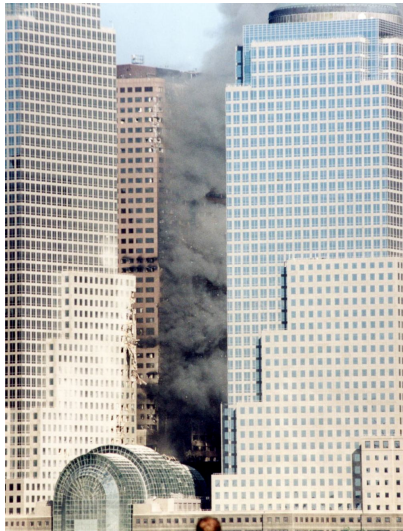
(Fig. 7) WTC 7 did produce some smoke towards the end of the day, but most of it came from WTC 6. Smoke hugging the face of WTC 7 creates the illusion that the building was fully involved.
